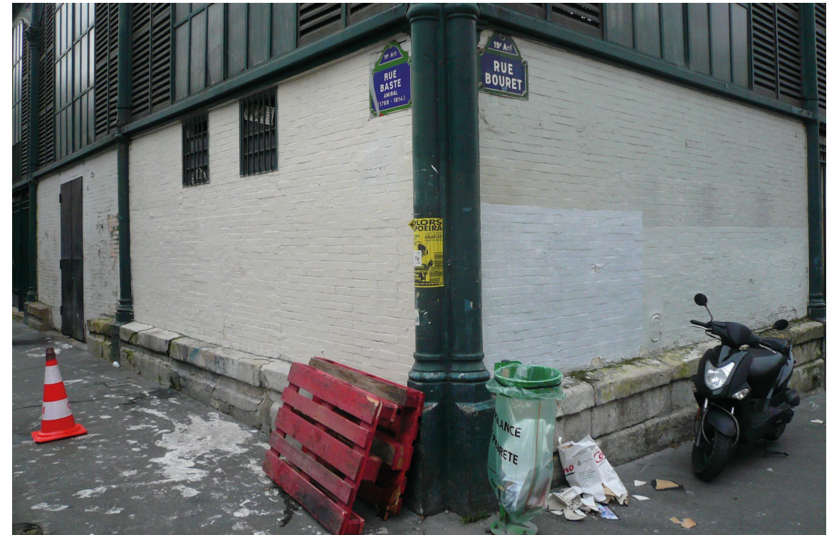
Etat avant restauration Condition prior to restoration works
