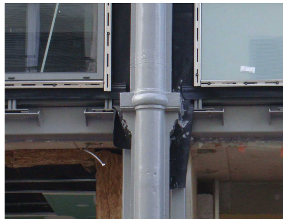
Installation des murs rideaux Installation of curtain walls
