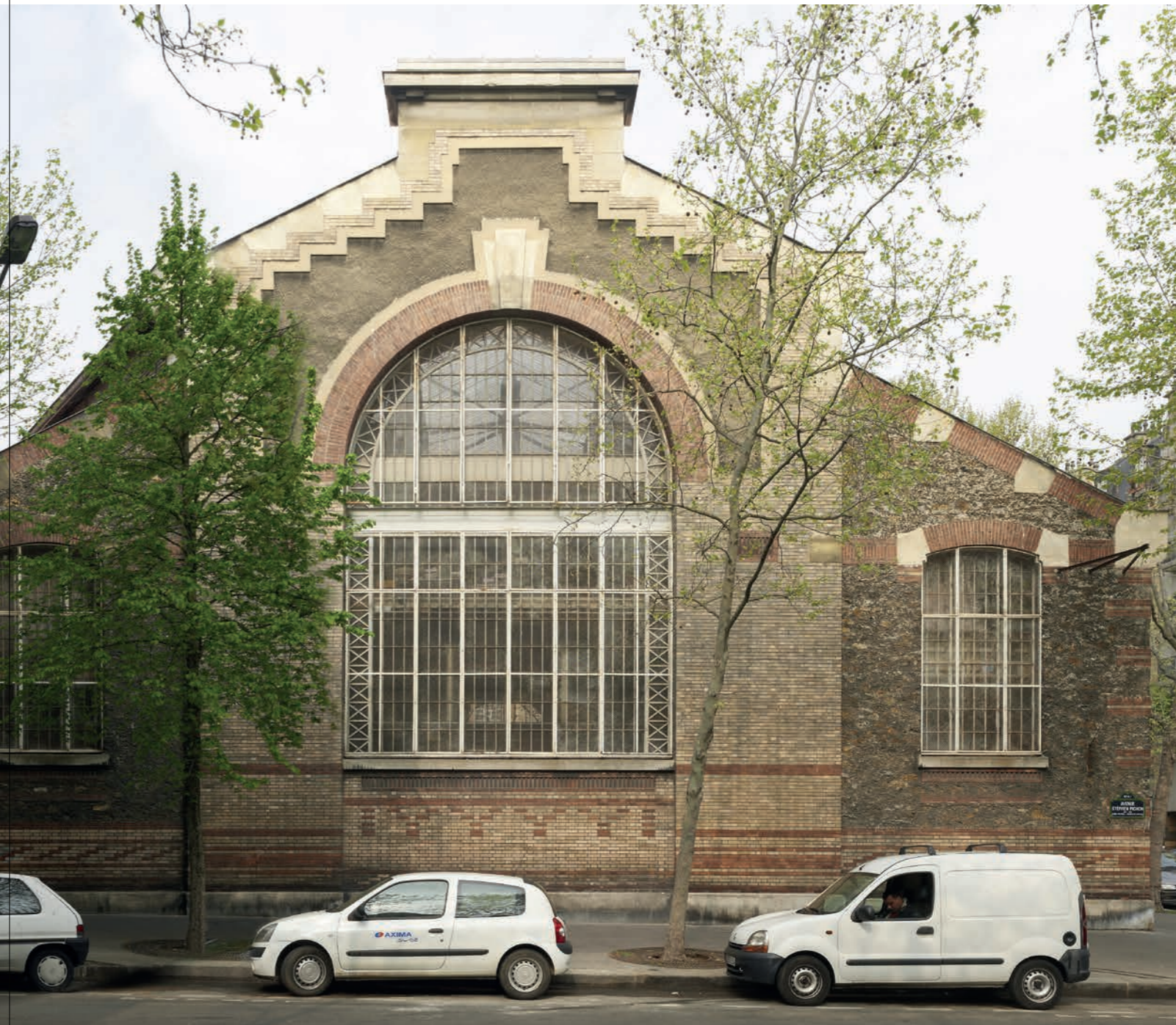
Research halls prior to works
